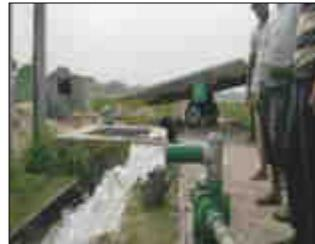
Solar operated centrifugal pump
